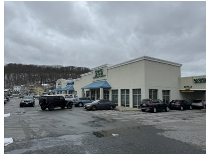
EXISTING VIEW FROM PARKING
